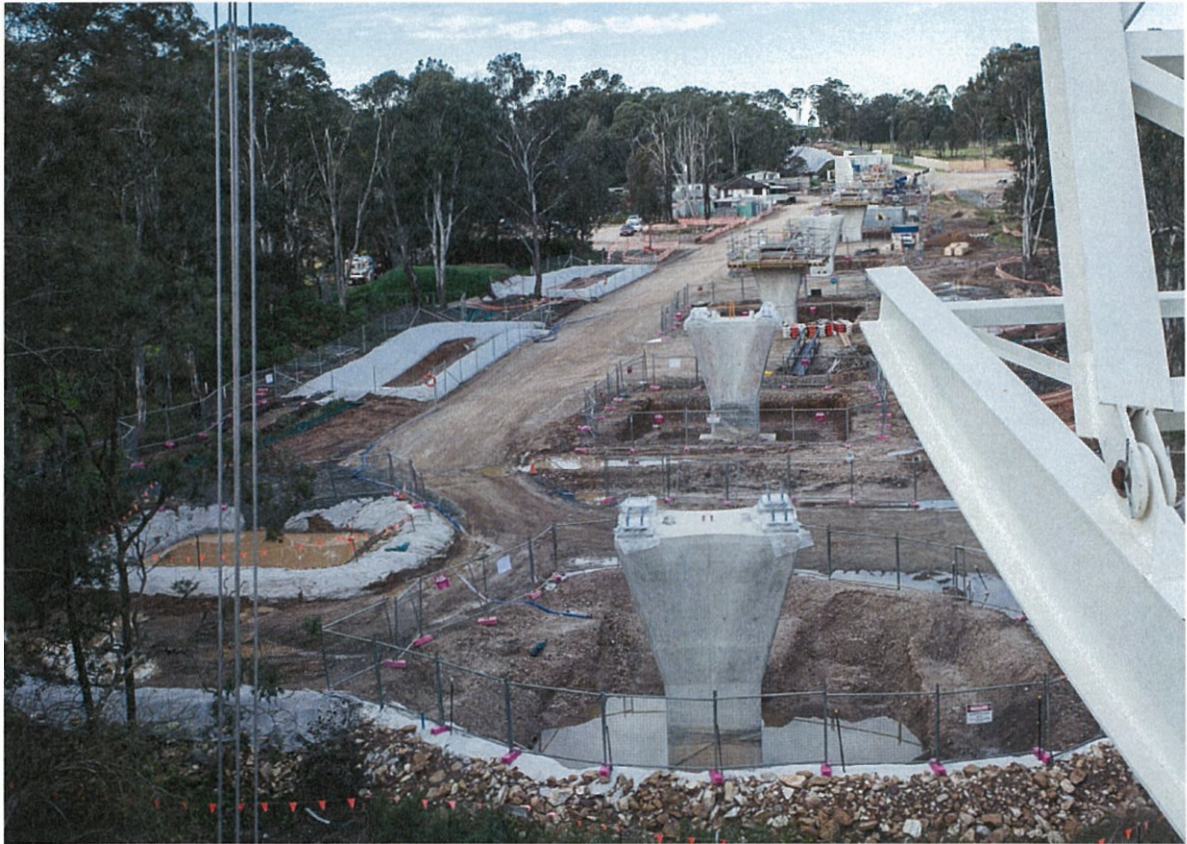
Figure 10 - Erosion and Sediment Controls at the Cudgegong Rd Site
