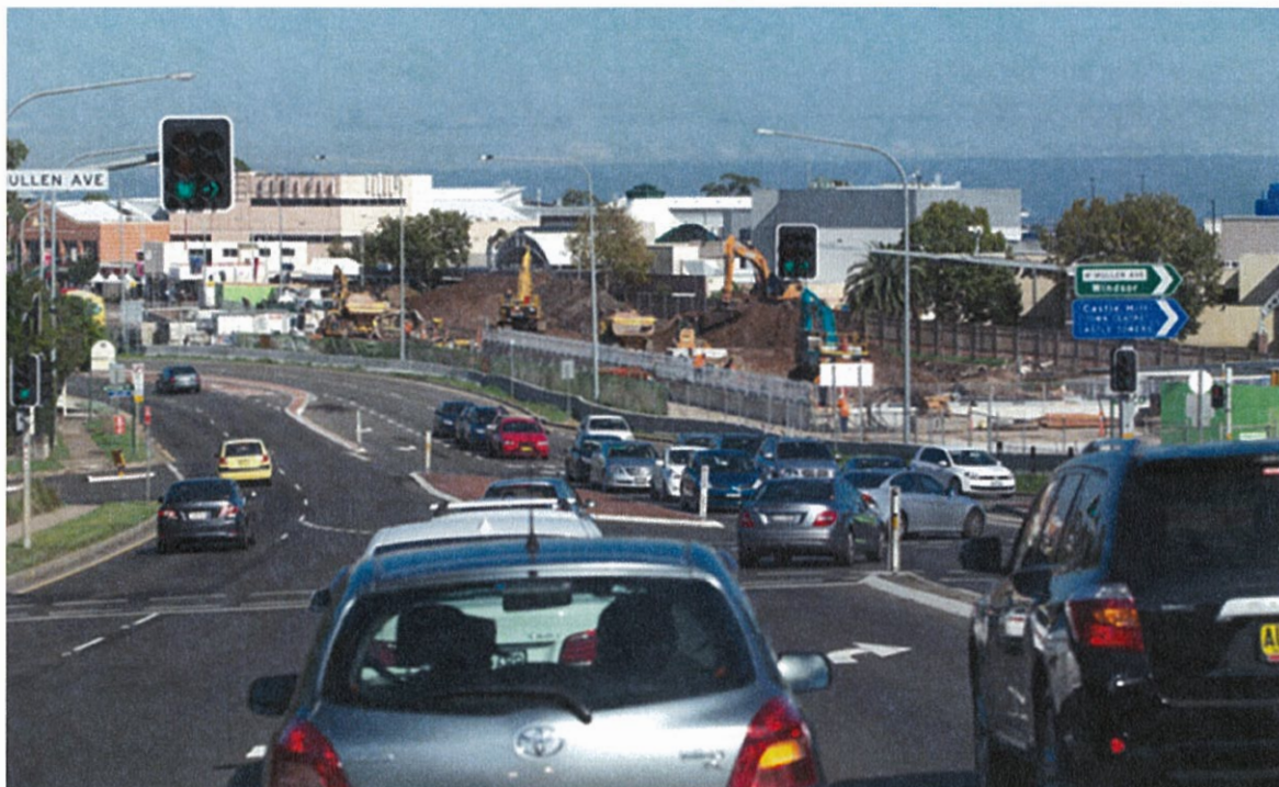
Figure 5 - Castle Hill Station Site at the Intersection of Old Northern Rd and McMullen Ave
