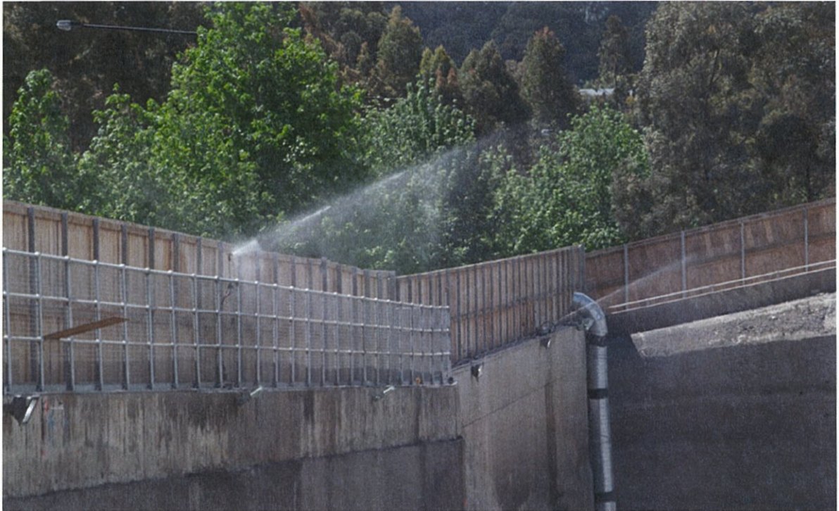
Figure 11 - Dust Mitigation at Norwest Station Site
