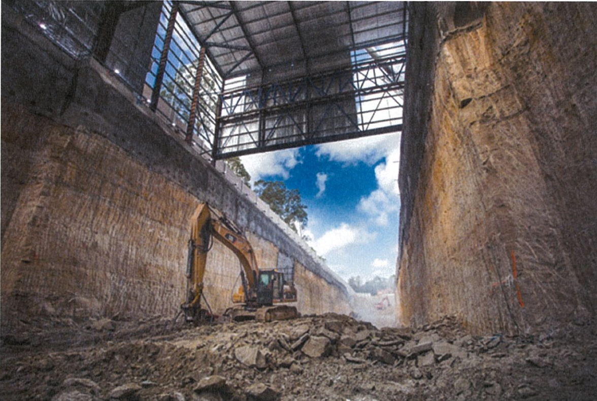
Figure 4 - Spoil and Excavation Works at the Showground Station Site
